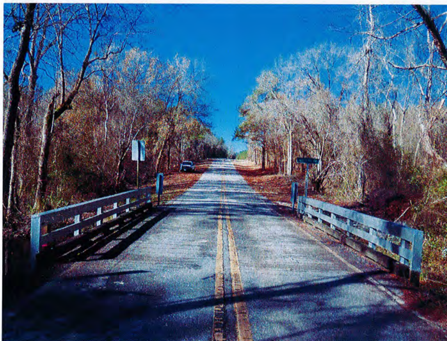
Photograph No. 2: This photograph was taken from the East approach of the -L- alignment, looking West
